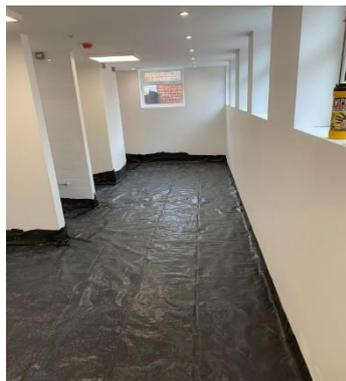
You should end up with a waterproof area, free of holes or gaps for the screed to escape. Screed working its way underneath insulation or membrane will result in all your efforts floating to the top of your screed.
