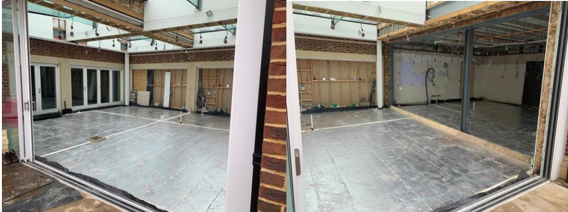
Now that your floor insulation is installed, it's time to install your top tanking membrane, this will create the final watertight layer between the insulation and/or sub-floor and your screed. **DO NOT STAPLE ANY UNDERFLOOR HEATING PIPES UNTIL THIS MEMBRANE IS INSTALLED. IF WE ARRIVE ON SITE AND YOU DON'T HAVE THIS MEMBRANE UNDERNEATH YOUR UNDERFLOOR HEATING PIPES, WE WOULD NOT BE ABLE TO INSTALL THE SCREED AND CANCELLATION CHARGES AS STATED IN OUR T'S & C'S WOULD APPLY.**
