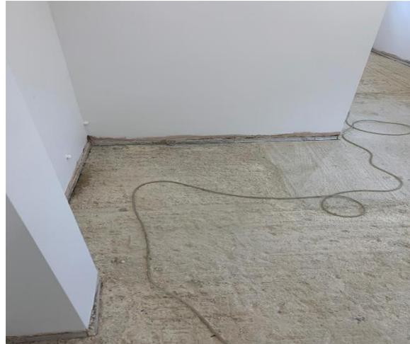
Now you need to go about tanking the sub-floor. Use a minimum 1000 Gauge DPM and spread the DPM(s) across the sub floor, making sure that all joints are taped. Ensure that the DPM is pushed tightly down to the wall base and lap the membrane up the walls or stud work around 5-6" above your finished floor datum. Make sure that all internal and external corners are pushed in tight and neatly folded (imagine you are wrapping a present!)
