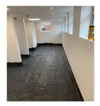
You should end up with a waterproof area, free of holes or gaps for the screed to escape. Screed working its way underneath insulation or membrane will result in all your efforts floating to the top of your screed.
