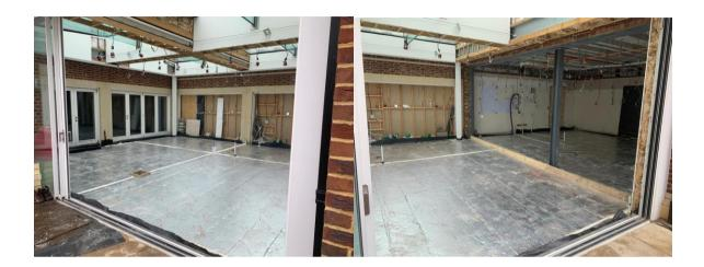
Now that your floor insulation is installed, it's time to install your top tanking membrane, this will create the final watertight layer between the insulation and/or sub-floor and your screed. DO NOT STAPLE ANY UNDERFLOOR HEATING PIPES UNTIL THIS MEMBRANE IS INSTALLED. IF WE ARRIVE ON SITE AND YOU DON'T HAVE THIS MEMBRANE UNDERNEATH YOUR UNDERFLOOR HEATING PIPES, WE WOULD NOT BE ABLE TO INSTALL THE SCREED AND CANCELLATION CHARGES AS STATED IN OUR T'S & C'S WOULD APPLY.
