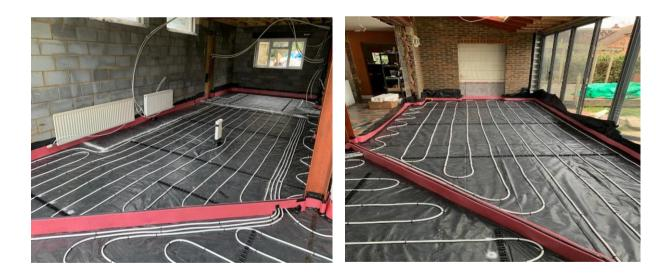
Make sure once your preparation is complete, that the area to be screeded is cleaned of dust and debris as this can compromise the finished look and texture of the floor.
